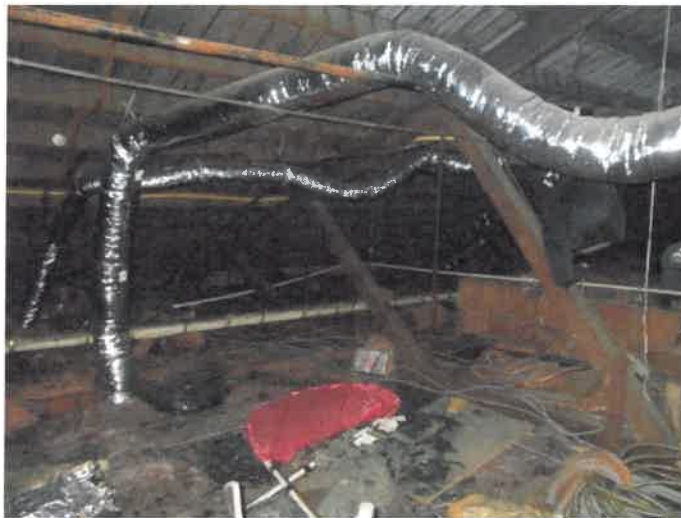
Figure 1. Roof Framing (Note Timber Truss and Roof Purlins)
