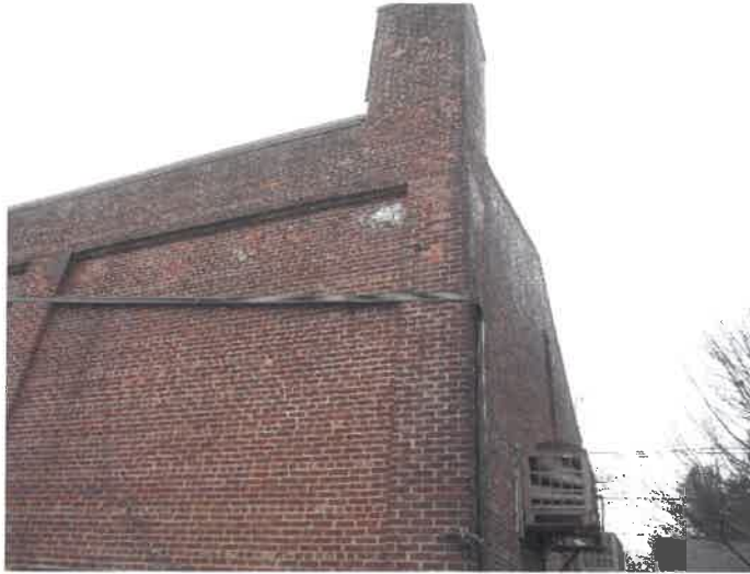
Figure 9. Notched Brick Masonry Piers to House Rain Leaders at South Elevation
