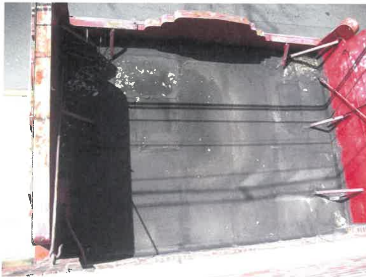
Figure 15. Overall View of Marquee Roof
