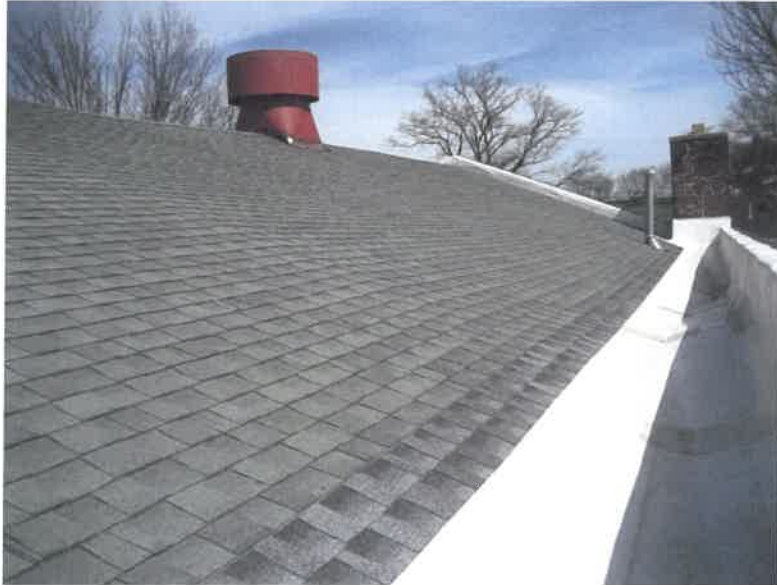
Figure 12. Overall View of Main Roof Area
