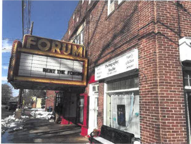
Figure 1. Front/West Elevation w/Marquee
