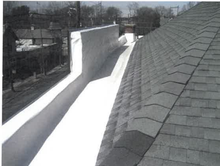
Figure 11. Overall View of Main Roof Area
