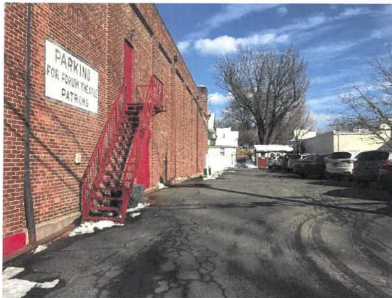
Figure 2. Right/South Elevation w/Exterior Metal Egress Stair
