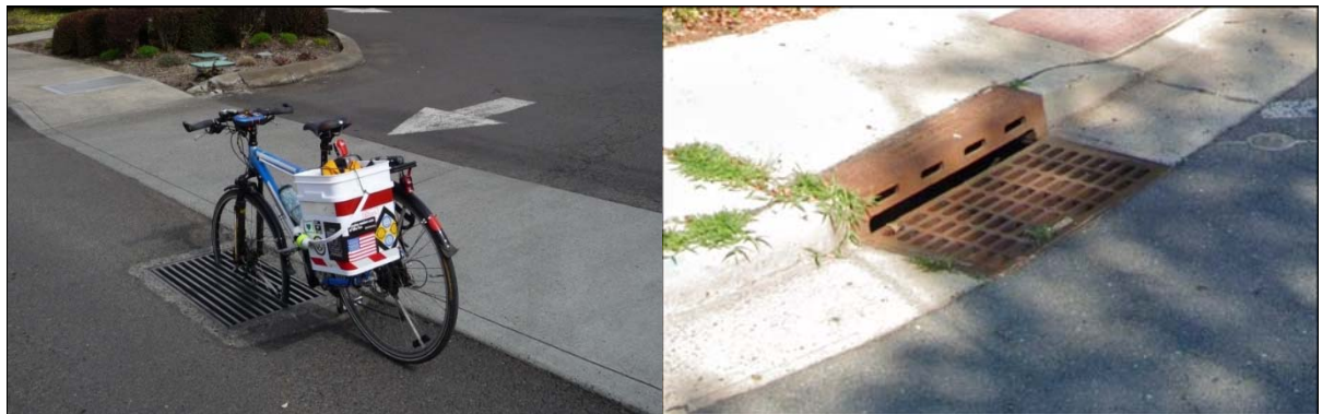
Example of a Non-Bicycle Safe Grate Image by KTesh licensed under Creative Commons.
