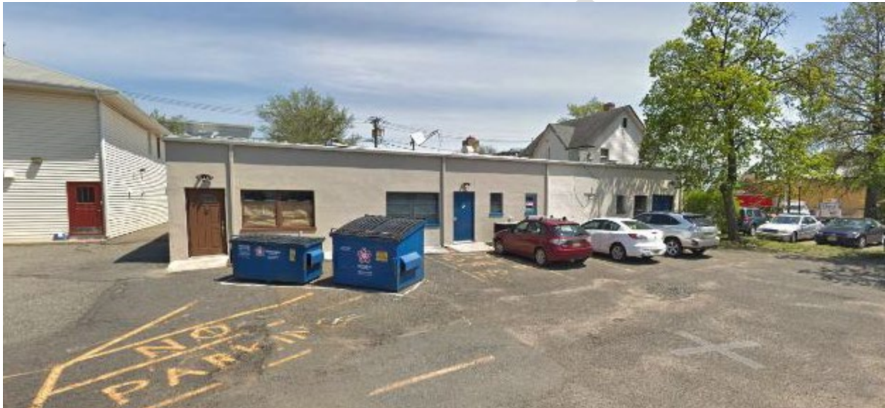
Figure 9. Google Street View of rear parking area, which has since been repaved.
