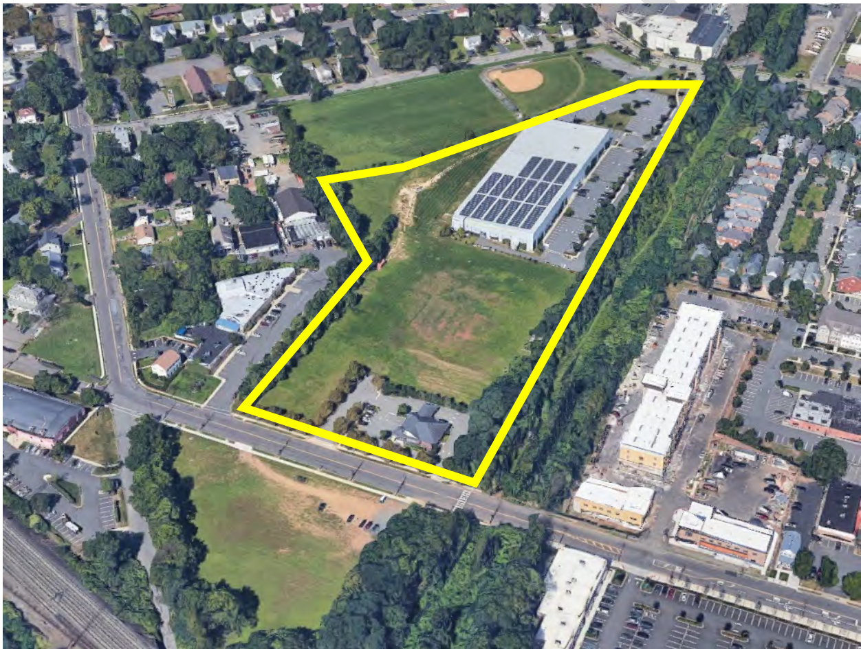
Bird's eye view of the Project Area, looking northwest, outlined in yellow. Source: Google Maps; screen capture on January 20, 2021. The Project Area is bounded by Middlesex Avenue with Trailhead Park beyond (bottom), Future Middlesex Greenway Extension (right) and Vidas Park (top).
