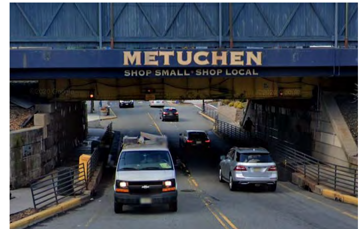
AMTRAK NEC Underpass
