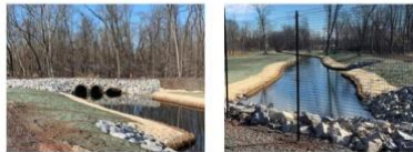
Environmental remediation of the property nearing completion
