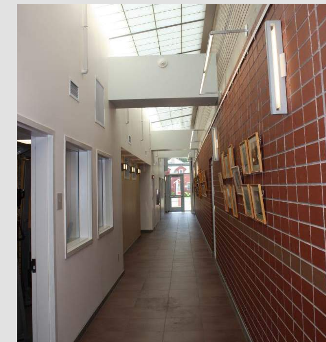
An interior corridor uses gel-insulated roof panel to allow dimmed light fixtures in the daytime. Electrical system incorporates roof photovoltaics.
