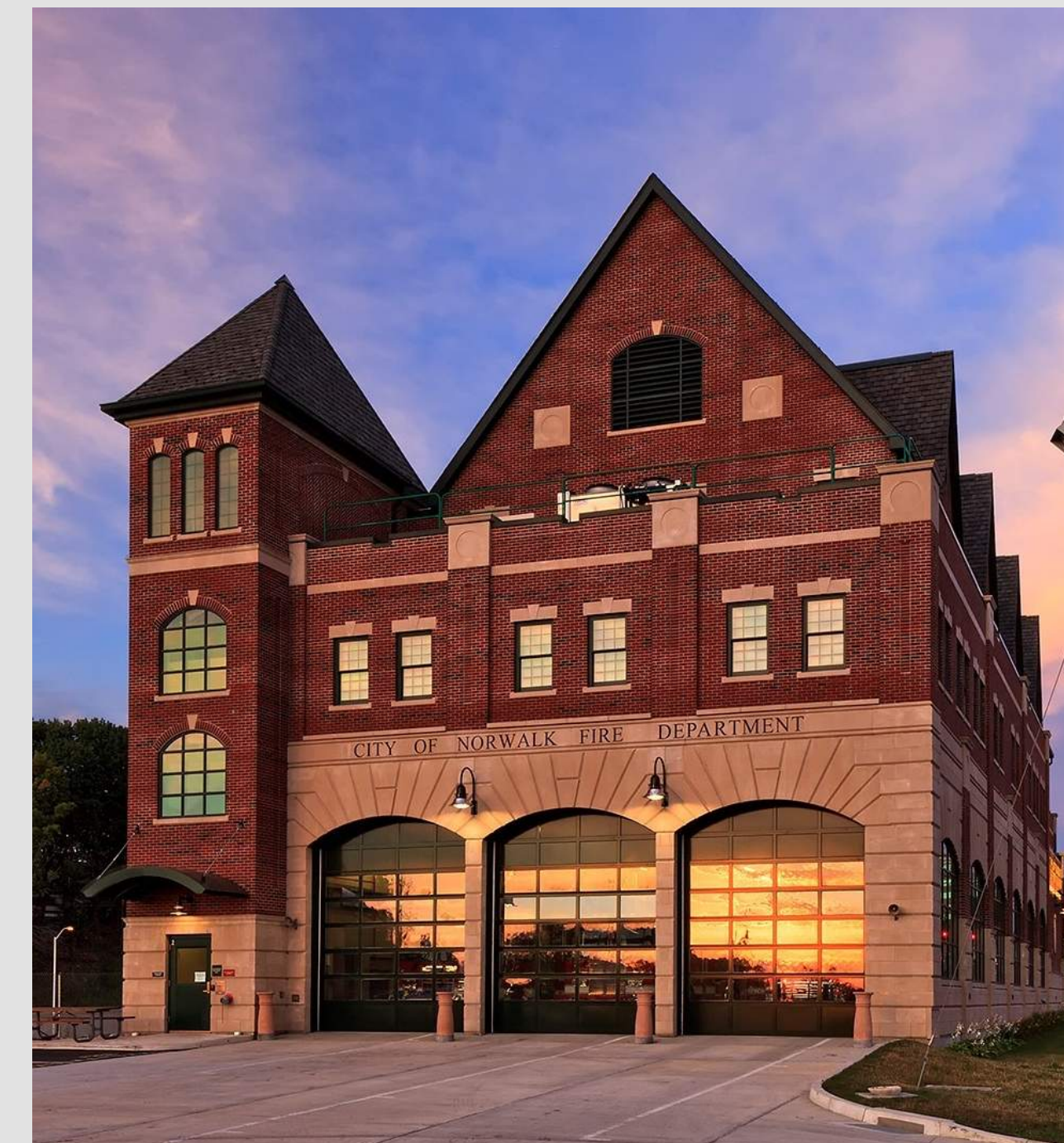
LEED Gold certification, Norwalk HQ uses a Variable Refrigerant Flow (VRF) mechanical system that allows personalized individual zone control and superior energy efficiency by internally harvesting and redistributing solar gain and other heat differentials in all seasons.
