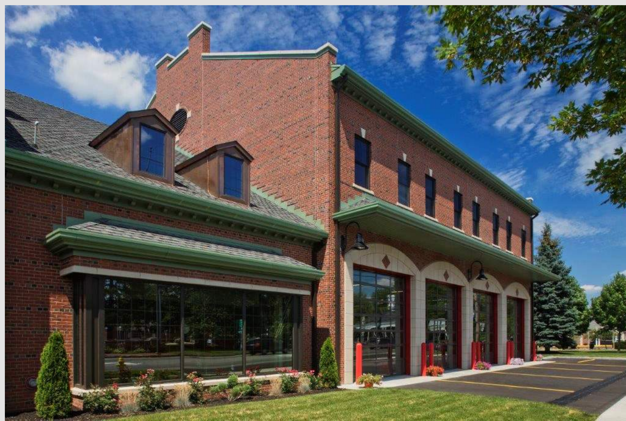
The Village of Fayetteville Fire Department is the first LEED Silver Fire Station in New York State.
