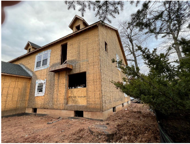
Left Side of House #2 (from rear angle)
