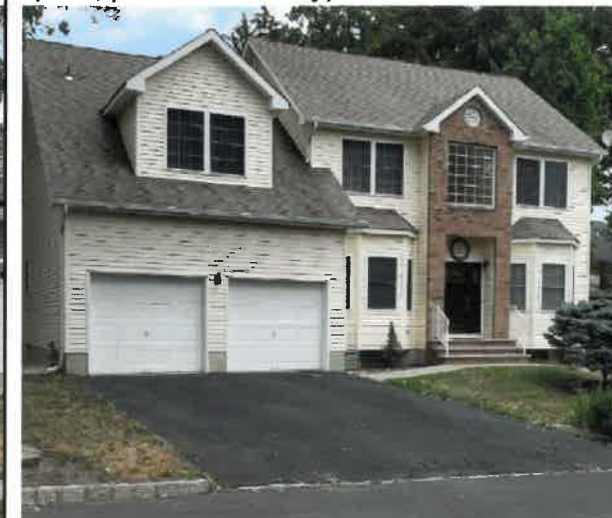
2 Wilson Lane (double wide driveway and apron; path to driveway)
