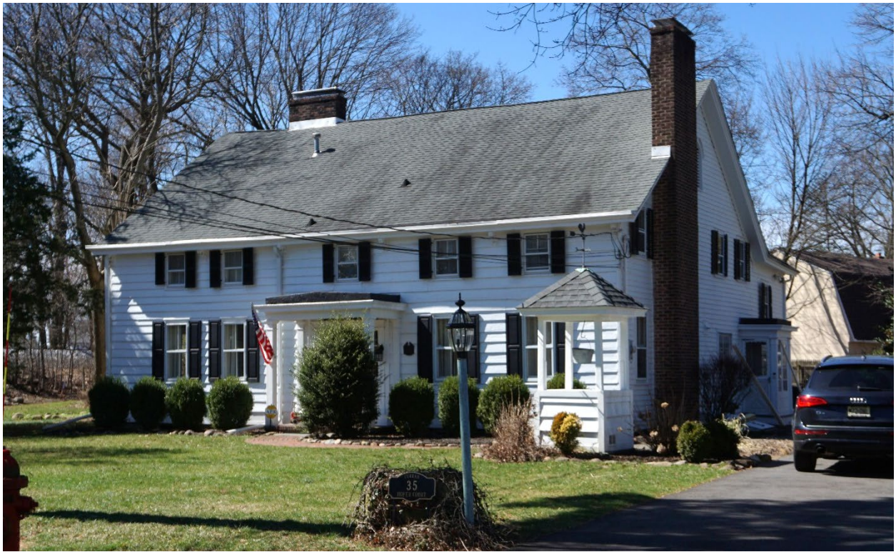
Photograph 10: Ross House at 35 Hofer Court
