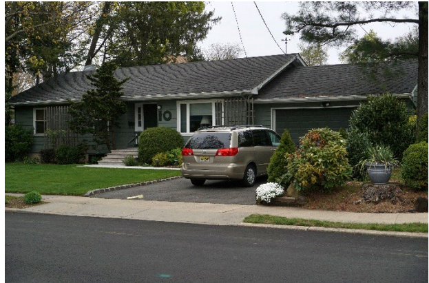
Photograph 29. Example of Ranch style
