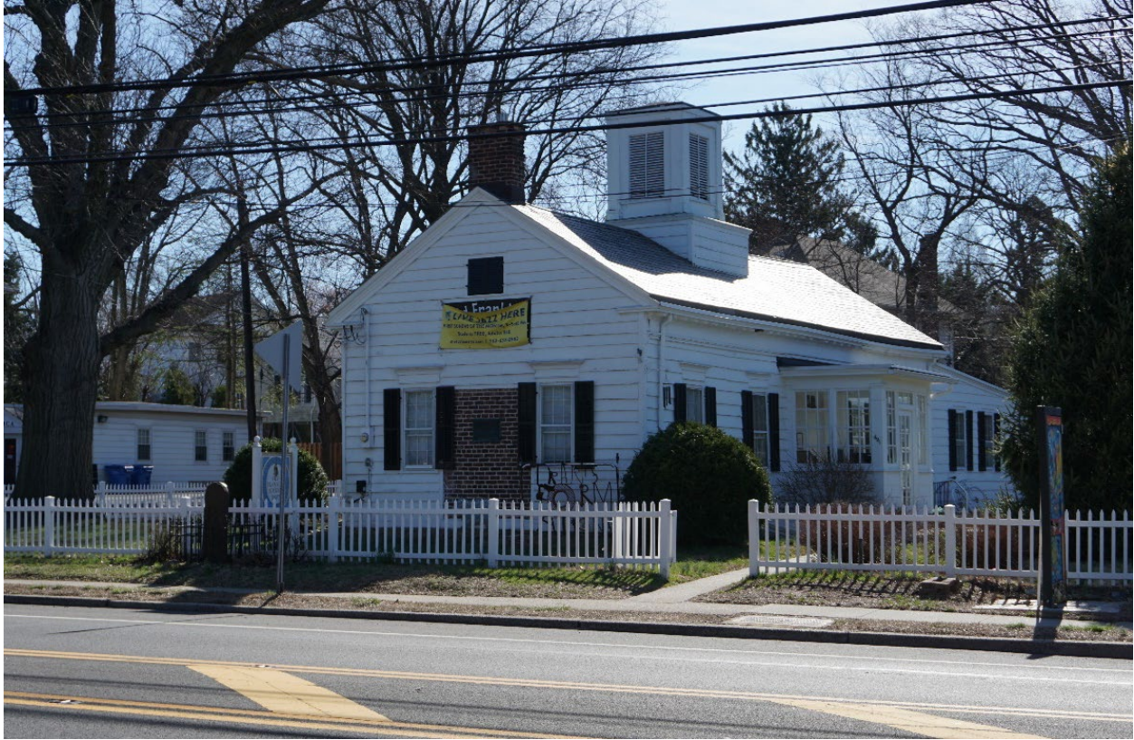
Photograph 5. Old Franklin Schoolhouse
