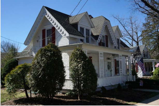
Photograph 13. Example of Gothic Revival style
