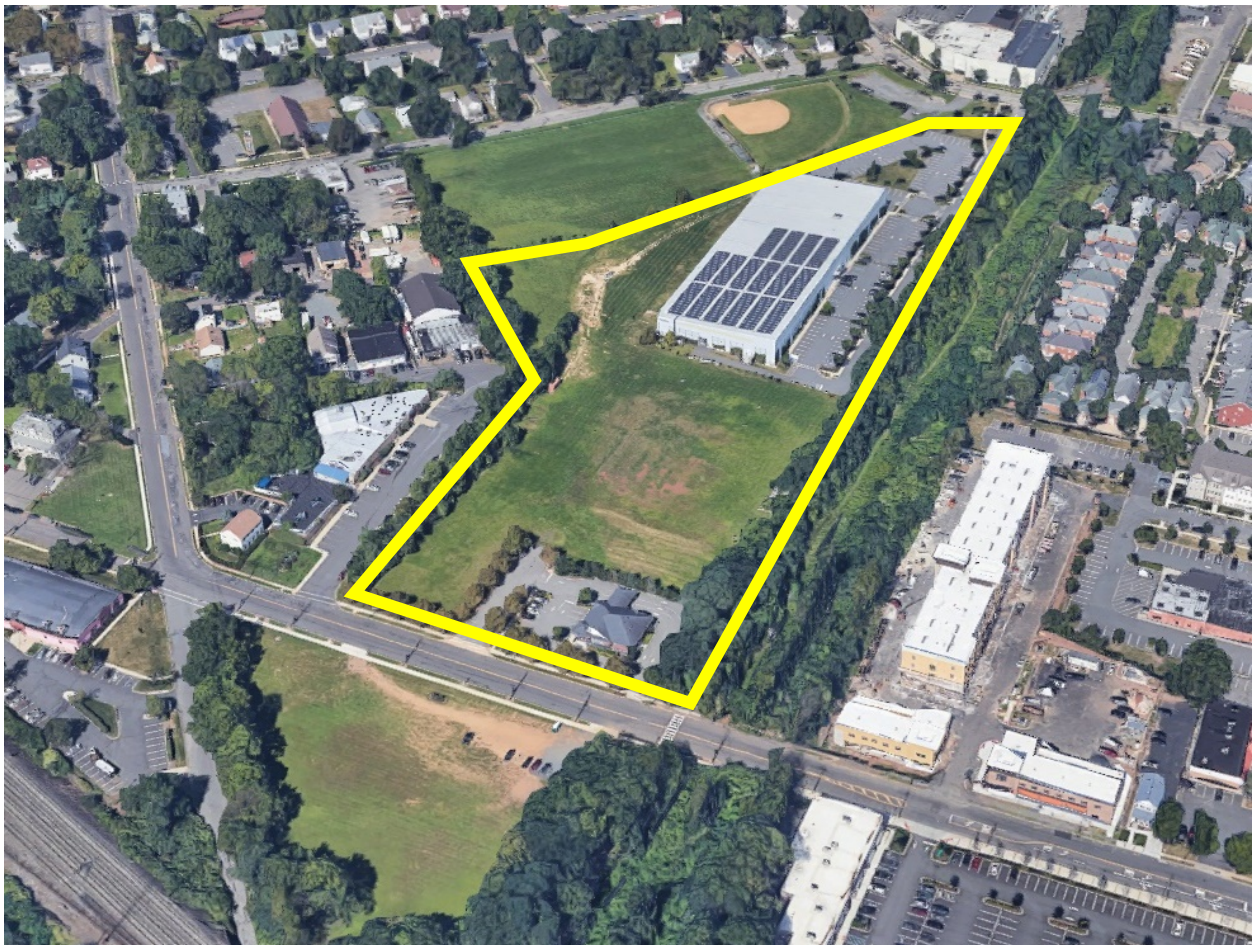
Bird’s eye view of the Project Area, looking northwest, outlined in yellow. Source: Google Maps; screen capture on January 20, 2021. The Project Area is bounded by Middlesex Avenue with Trailhead Park beyond (bottom), Future Middlesex Greenway Extension (right) and Vidas Park (top).
