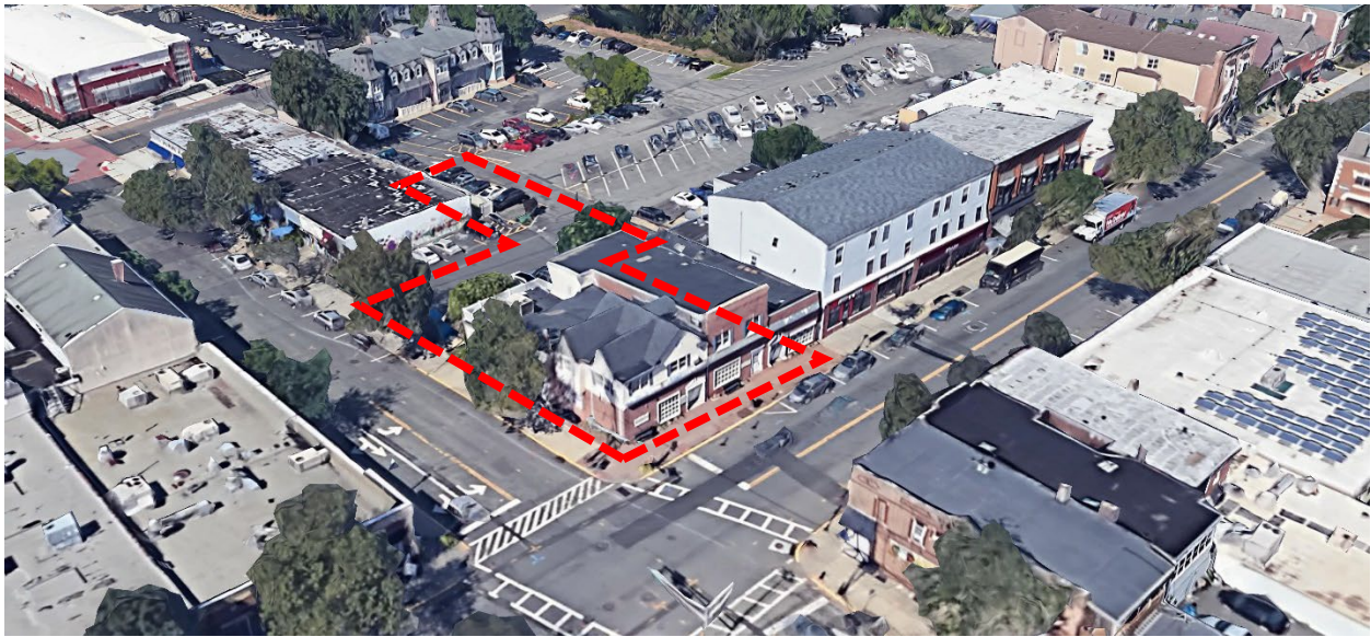
Figure 13. Bird's eye view of Project Area #2, looking northwest, outlined in red. Source: Google Maps; screen captured on July 27, 2020.
