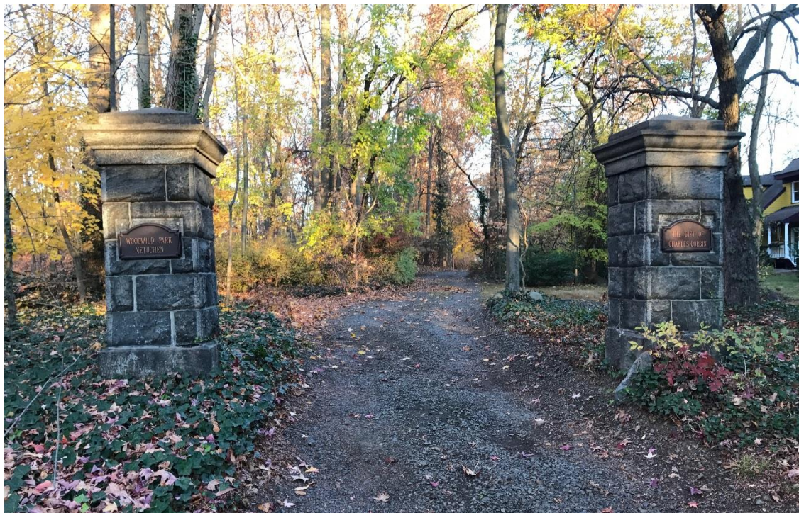
Photograph #04. Woodwild Park stone entrance columns. November 18, 2016, Michele Clancy.
