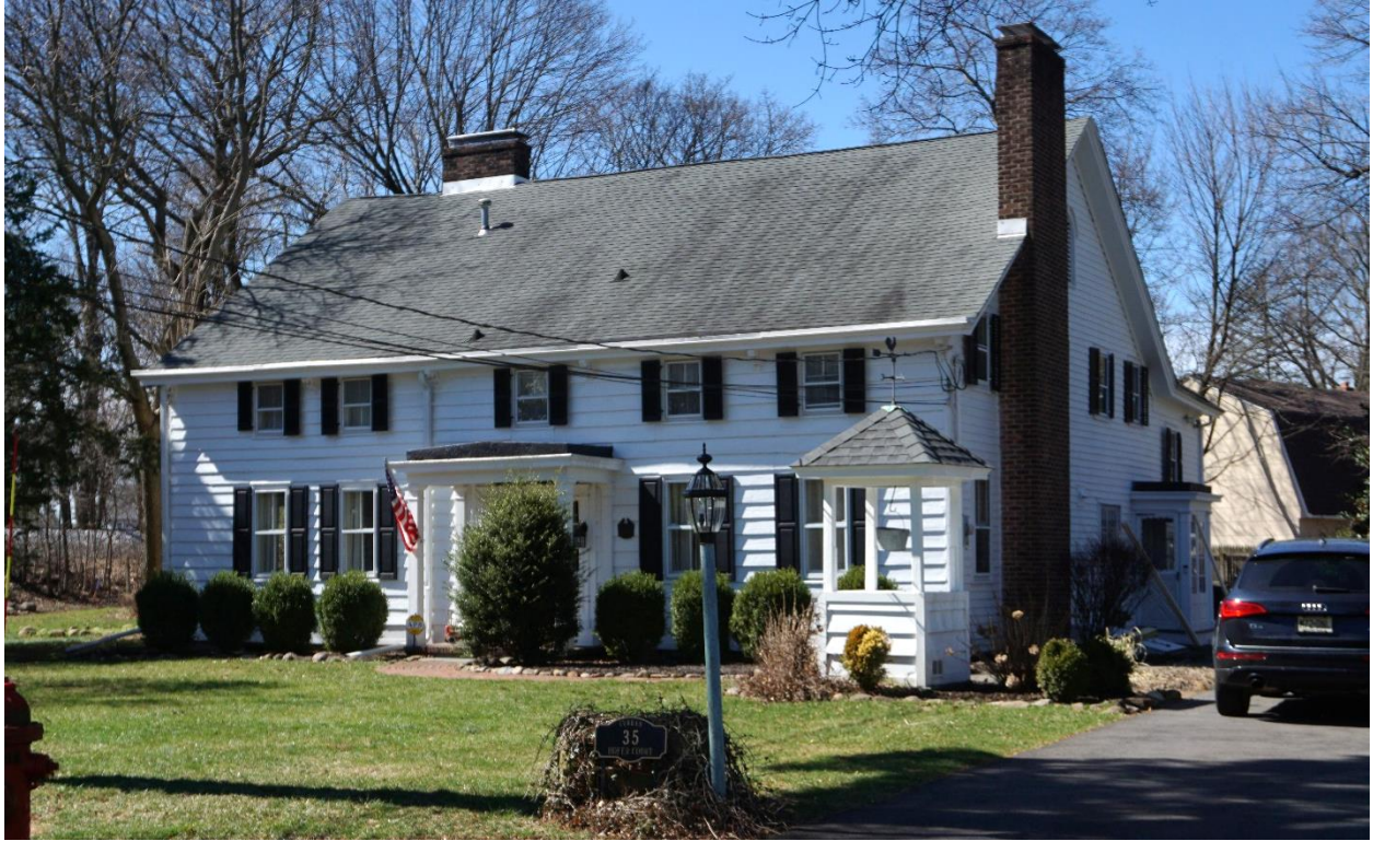
Photograph 10: Ross House at 35 Hofer Court
