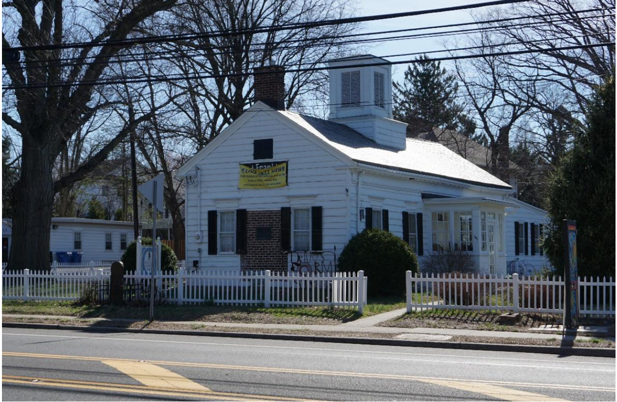
Photograph 5. Old Franklin Schoolhouse
