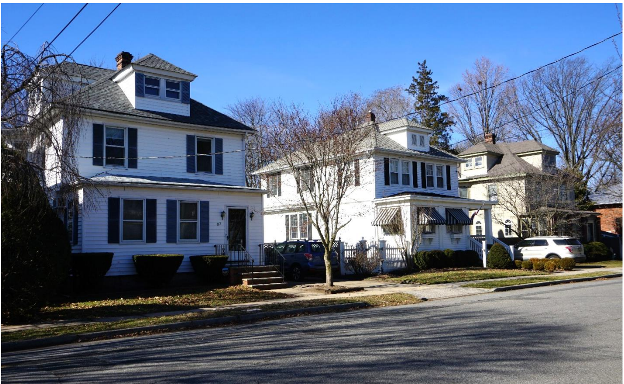
Photograph 21. Examples of American Foursquare style
