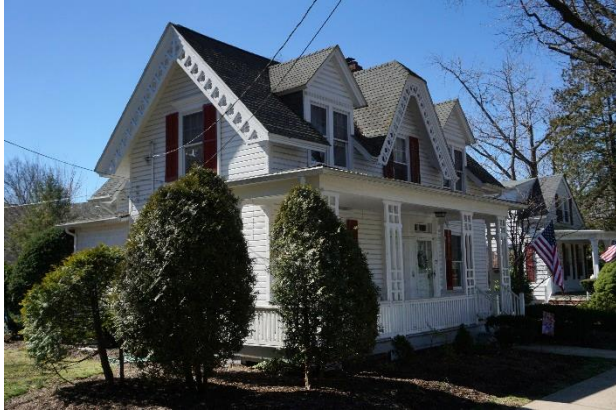
Photograph 13. Example of Gothic Revival style
