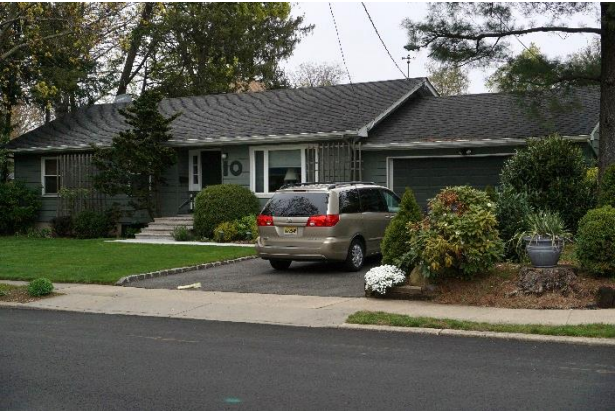
Photograph 29. Example of Ranch style
