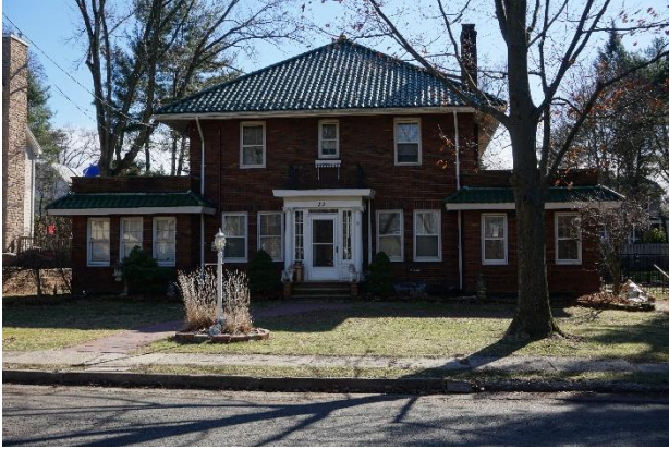
Photograph 22. Example of American Foursquare style
